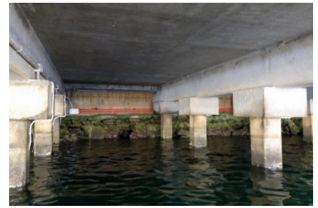
Desktop assessment identified and assessed remedial options for the wharf.
