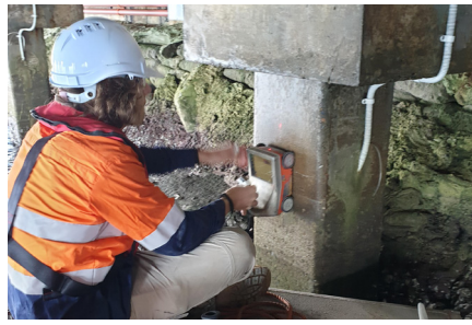
Testing on site as part of the investigation.
